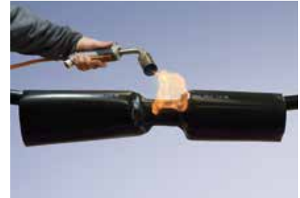
Apply the heat shrinkable tube
