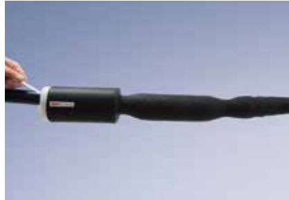
Apply the cold shrinkable tube
